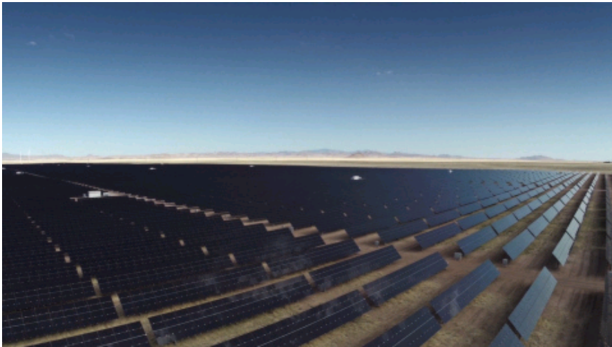
#1MachoSprings - Largest Solar Facility in New Mexico (Photo: Business Wire)
