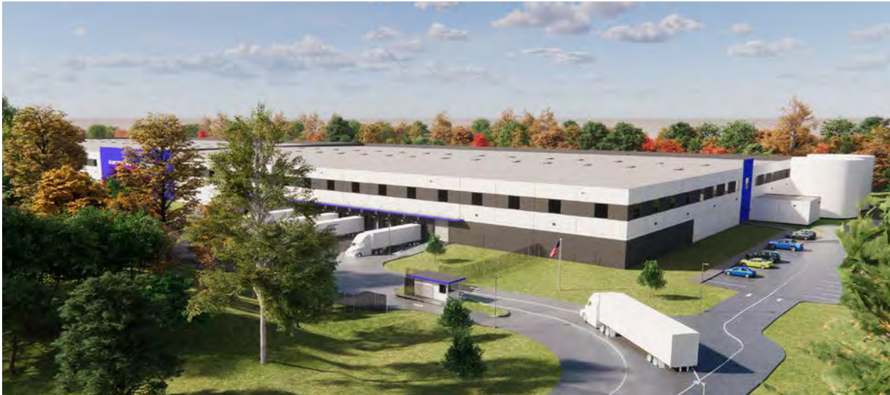
Electric Boat's new advanced warehouse and logistics center will improve environmental protection and reduce truck traffic by 80% at its Groton shipyard.
