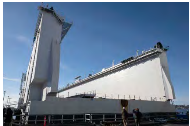
Floating dry dock at Electric Boat
