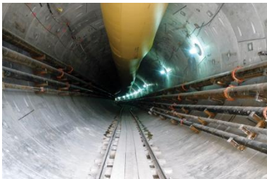
East Side Access Queens Tunnels, NY
