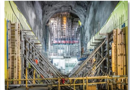
East Side Access Project, New York
