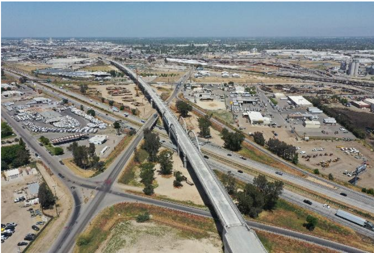
California High-Speed Rail CP1 Madera-Fresno, CA PROJECT VALUE: $4.0B
