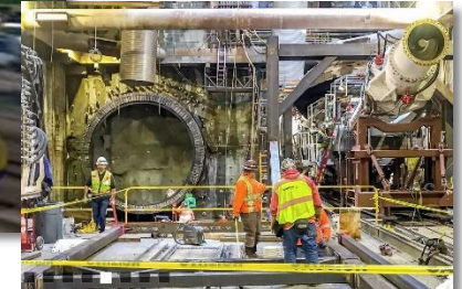
Purple Line Extension, Section 2, CA
