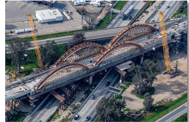
California High-Speed Rail Project, Central California
