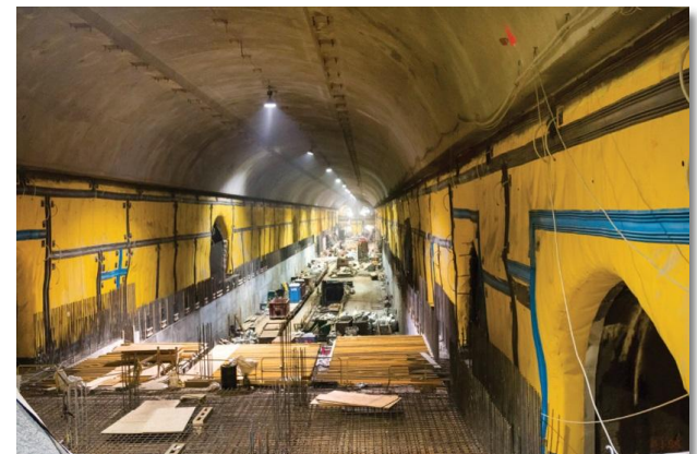
East Side Access Project, New York
