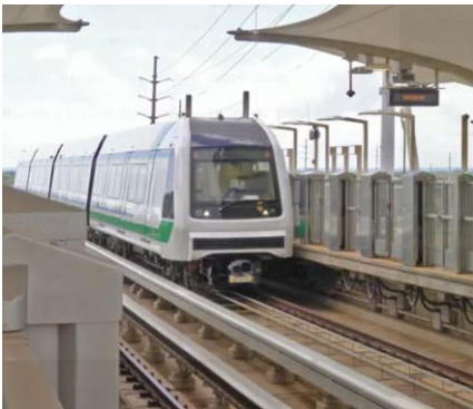
City Center Guideway & Stations, Honolulu
