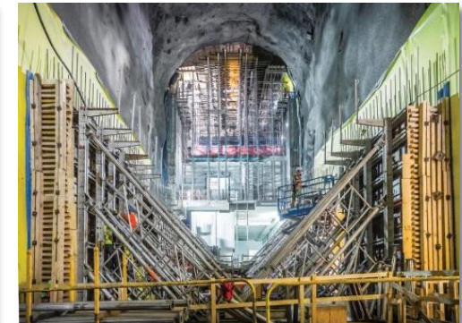
East Side Access Project, New York
