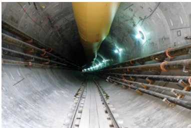
East Side Access Queens Tunnels, NY
