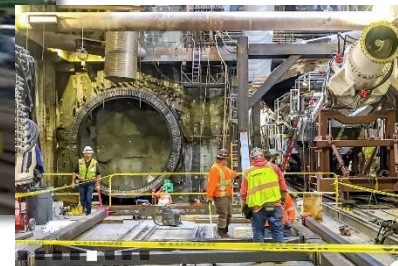
Purple Line Extension, Section 2, CA
