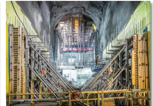
East Side Access Project, New York
