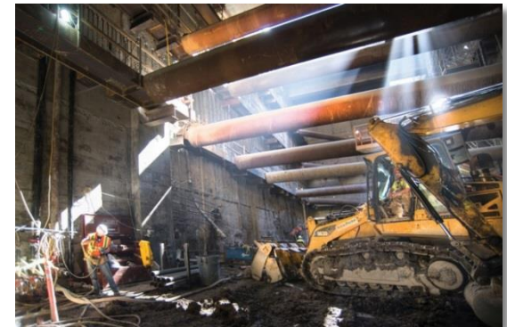
Central Subway T-Line Extension, San Francisco
