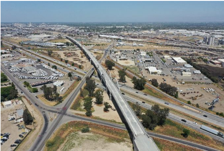
California High-Speed Rail CP1 Madera-Fresno, CA PROJECT VALUE: $3.9B
