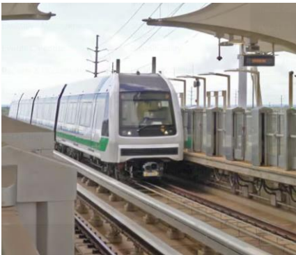
City Center Guideway & Stations, Honolulu
