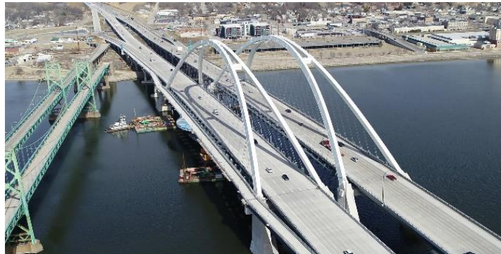
I-74 Mississippi River Bridge, Bettendorf, IA – Moline, IL
