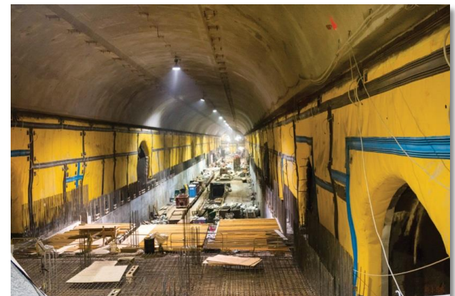
East Side Access Project, New York
