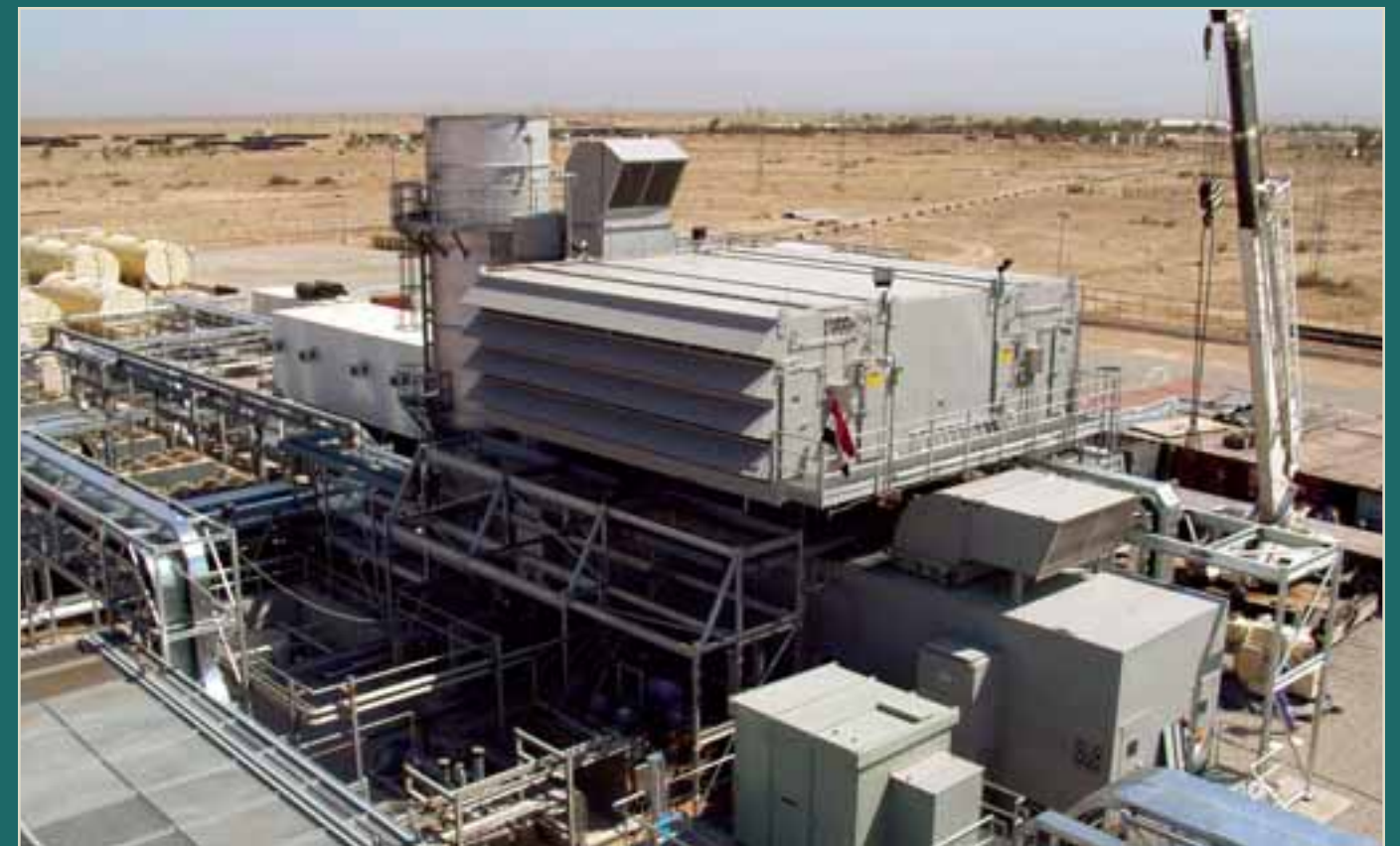
Below Right: Labor Crew on Break Electrical Infrastructure, Iraq
