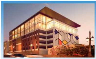
Maxwell | Redevelopment Los Angeles (Arts District) 102,963 SF | Completed 1Q19 Multi-Tenant
