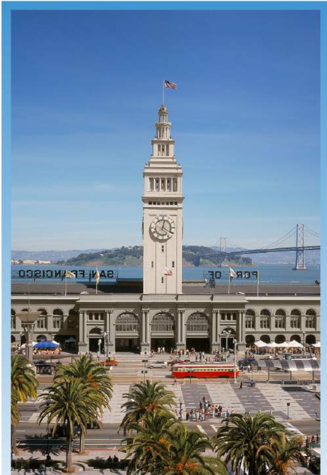
Ferry Building | San Francisco, CA
