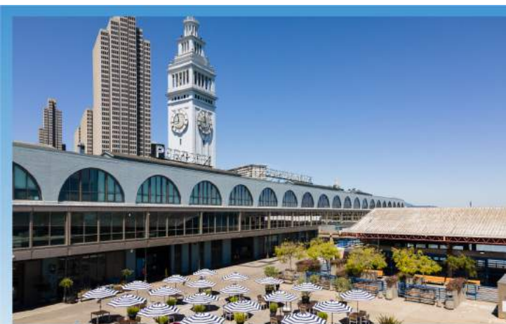
Ferry Building | San Francisco, CA
