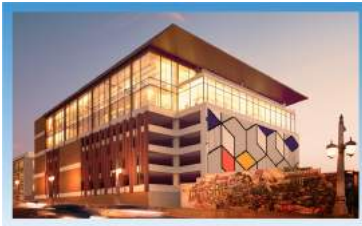
Maxwell | Redevelopment Los Angeles (Arts District) 102,963 SF | Completed 1Q19 Multi-Tenant
