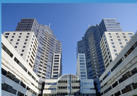
Rincon Center | San Francisco
