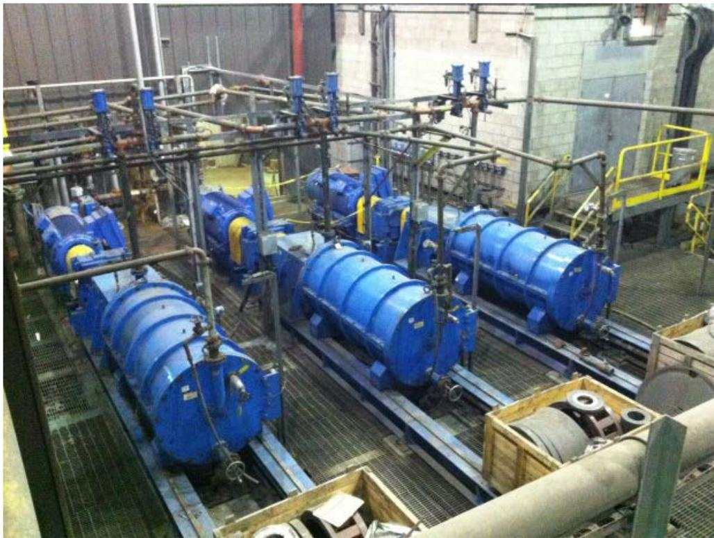
Figure 2: Three M1000 IsaMills installed at Trevali's Caribou mill
