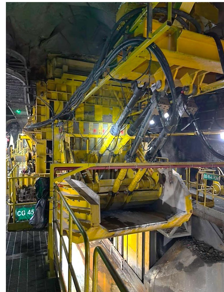
Installation of chute regulators continues on schedule
