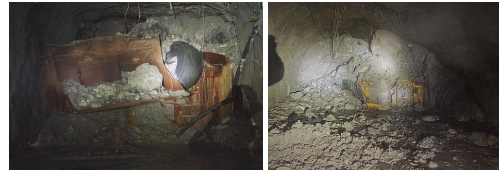
Buried LHD Loaders on Extraction Level, PB1C
