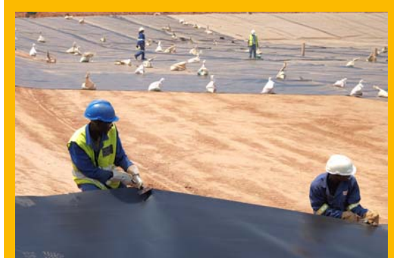
Workers install a liner for the Tailings Storage Facility
