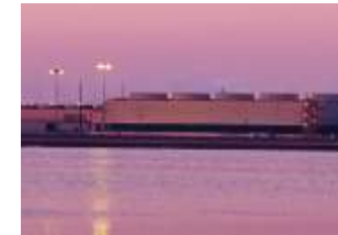
Salton Sea Geothermal 10 MW
