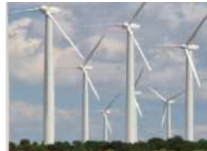
Aragonne Mesa Wind 90 MW
