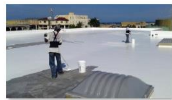
Liquid Applied Roofing
