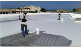
Liquid Applied Roofing
