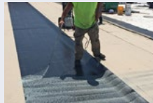
CAV-GRIP® III Low-VOC Adhesive/Primer A cold-weather adhesive with strong adhesion and low emissions
