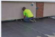
FleeceBACK® RL EPDM RapidLock® Membrane Fully adhered system offers long-term durability and ease of installation
