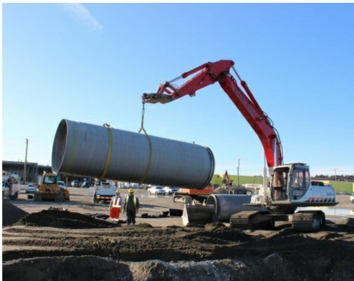
Delivered from the recently opened ADS distribution yard in Abbotsford, a 6-meter (20-foot) long section of large diameter SaniTite HP pipe is moved into place for a nearby mega-mall project. (Photo: Business Wire)
