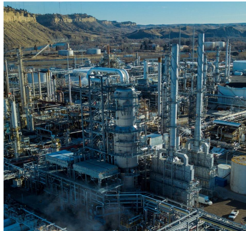
Vacuum Tower, Billings Refinery, Billings, MT
