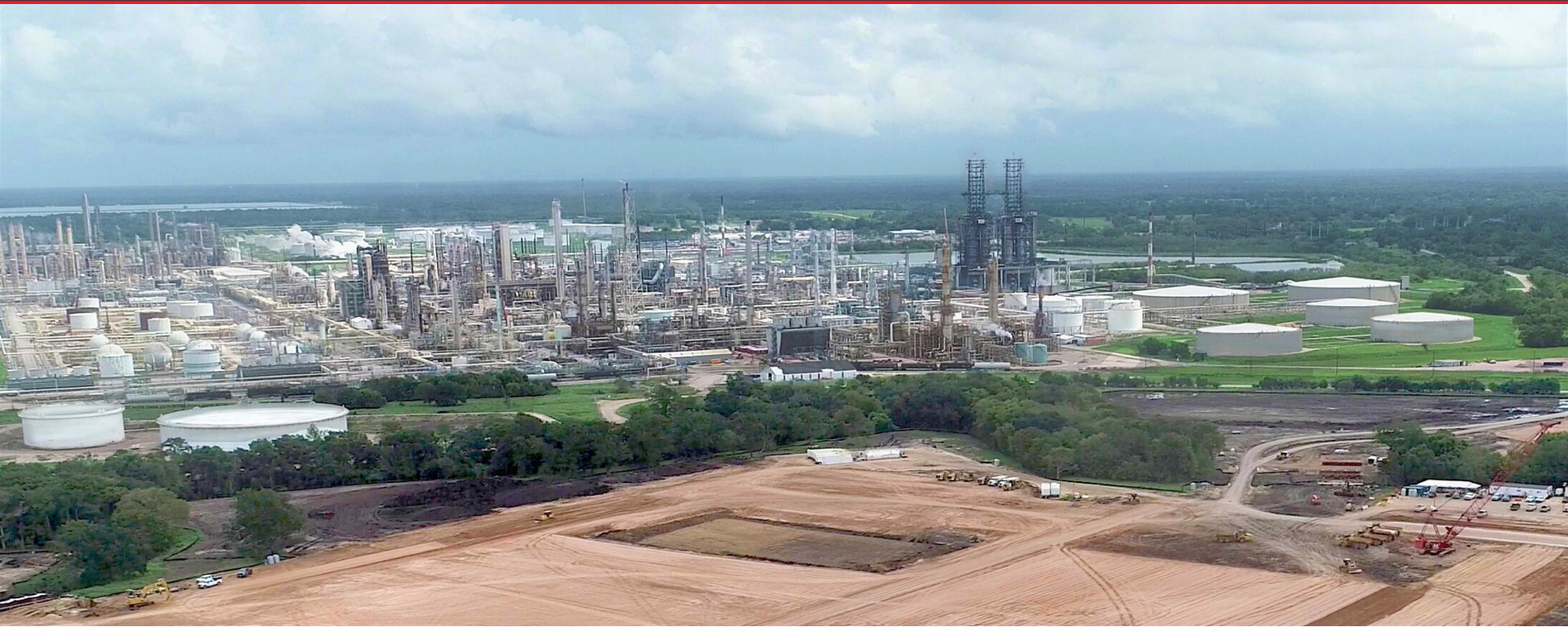
New fractionation site and Sweeny Refinery, Old Ocean, Texas
