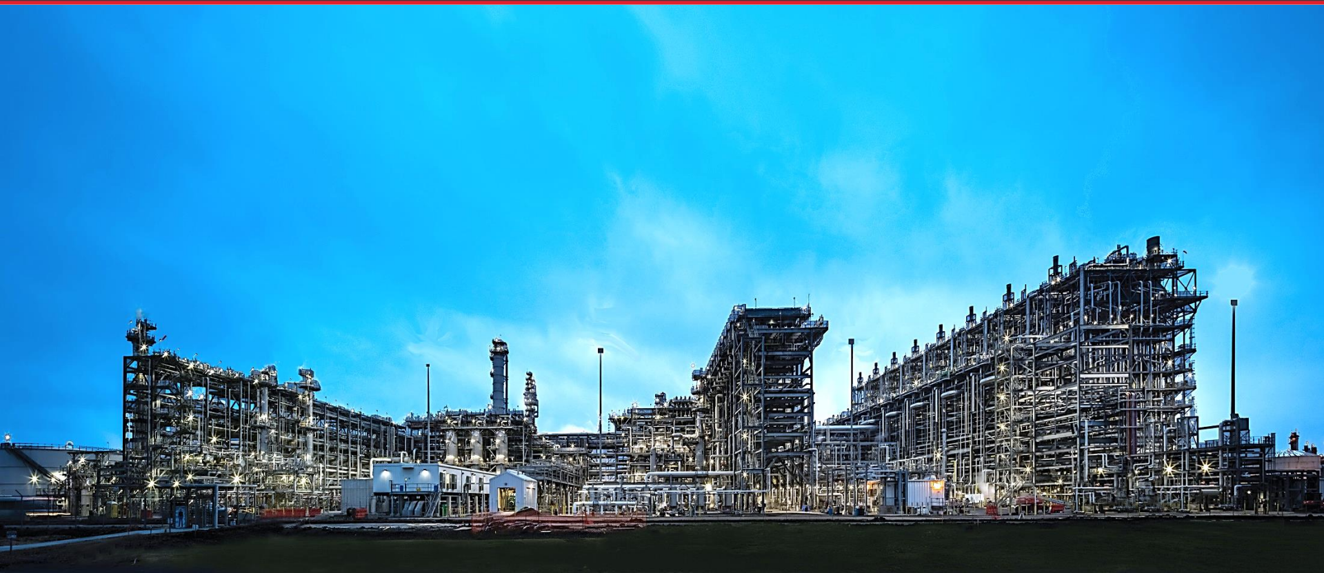
CPChem Cedar Bayou Facility, Baytown, Texas
