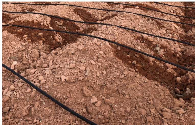
Figure 17-1, Leach Pad Surface
