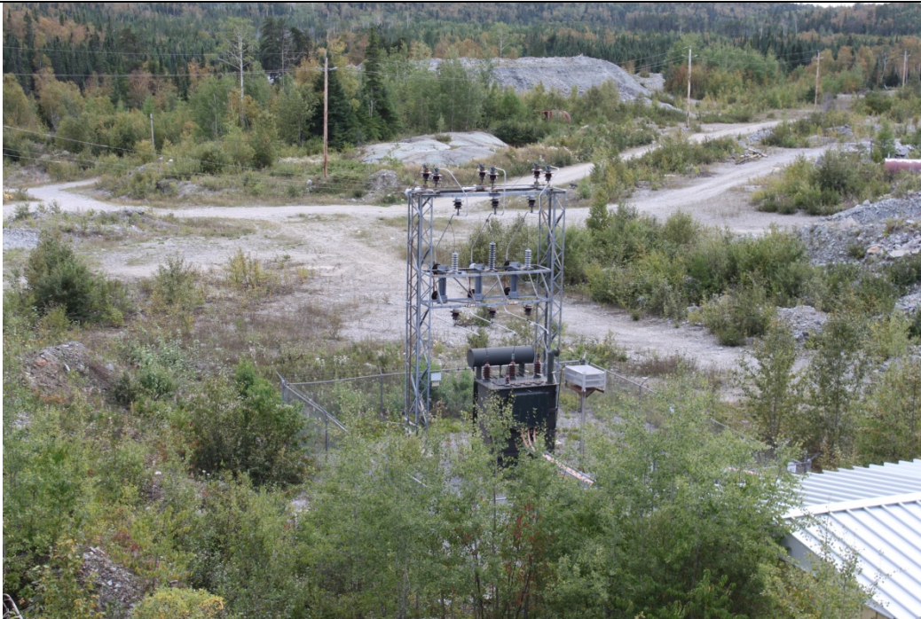
Picture 3 Existing Mine Site with Exploration Drills – Facing East (Project Pit)
