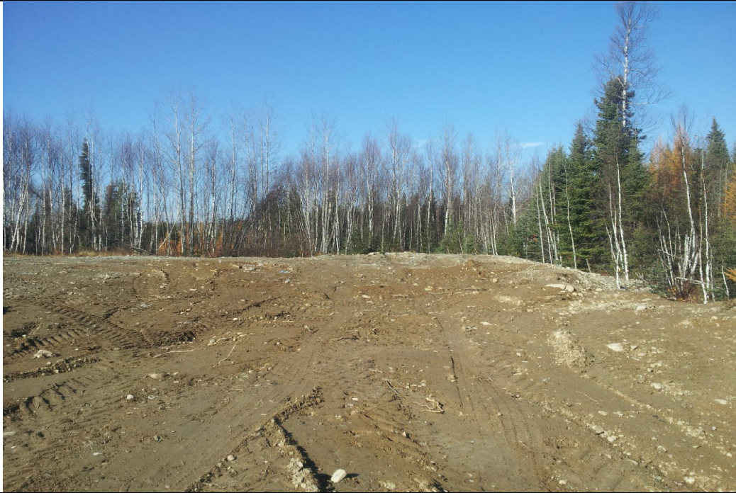
Picture 12 Existing Landfill Area - Facing North (Clean closed as part of Project)
