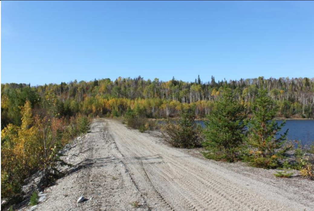
Picture 7(a) Existing Tailings Facility Centre Dam – Facing North (To be closed)
