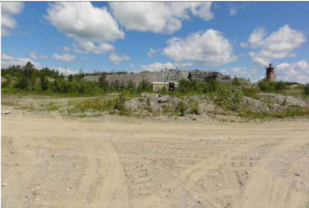
Picture 15 Looking Easterly Across Previous Mine Workings, North Shore of Webb Lake (Project Pit)
