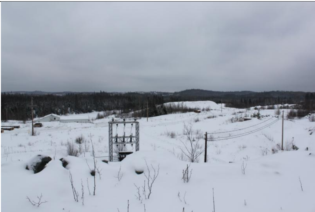
Picture 4 Existing Mine Site – Facing South (Project Pit)
