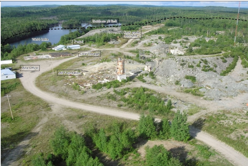
Picture 11 Existing Mine Facilities - Facing West (Project Pit)
