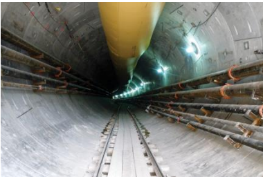
East Side Access Queens Tunnels, NY
