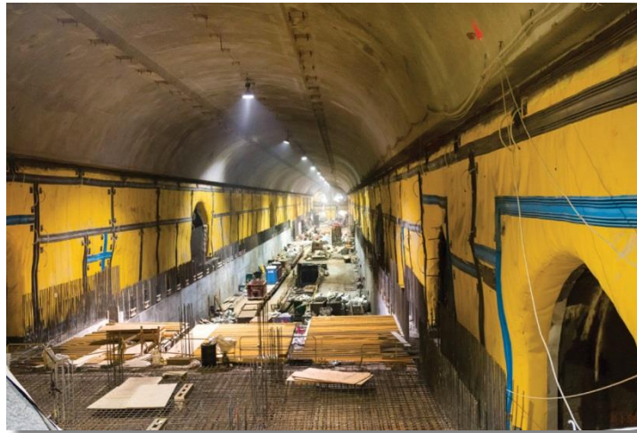
East Side Access Project, New York
