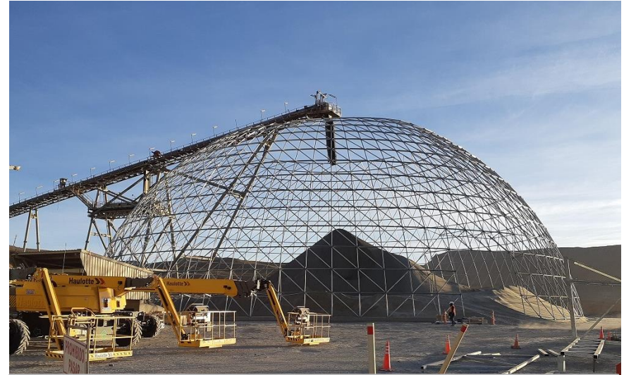
Stockpile dome construction – structural erection
