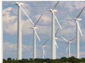
Aragonne Mesa Wind 90 MW
