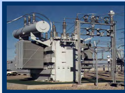
Remote switching Substation on-line monitoring Capacitor controls Distribution sensors
