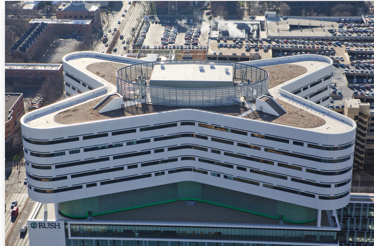
Carlisle TPO Roof - Rush University Medical Center in Chicago, IL
